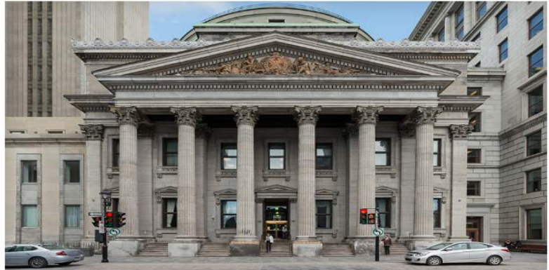
Bank of Montreal head office in Montréal. (Photo: DXR, via Wikimedia Commons)
